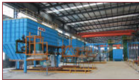
Vacuum sealed molding line
