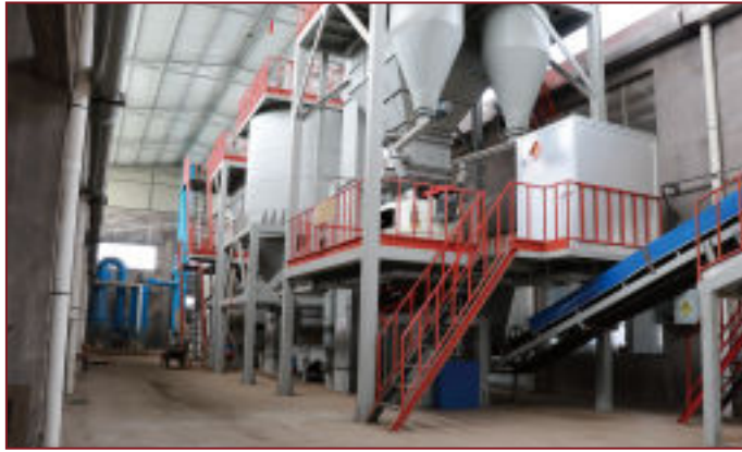
Green Sand Reclamation Production Line
